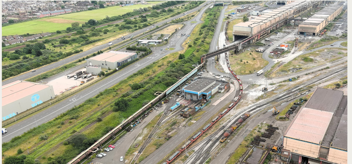
The snakelike 25 wagons carrying around 2.3KT of slab into Port Talbot in what will be daily deliveries for the next three years until the EAF is up and running
