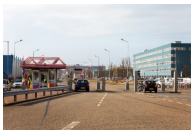
TATA MAIN GATE AT ROOSWIJK
