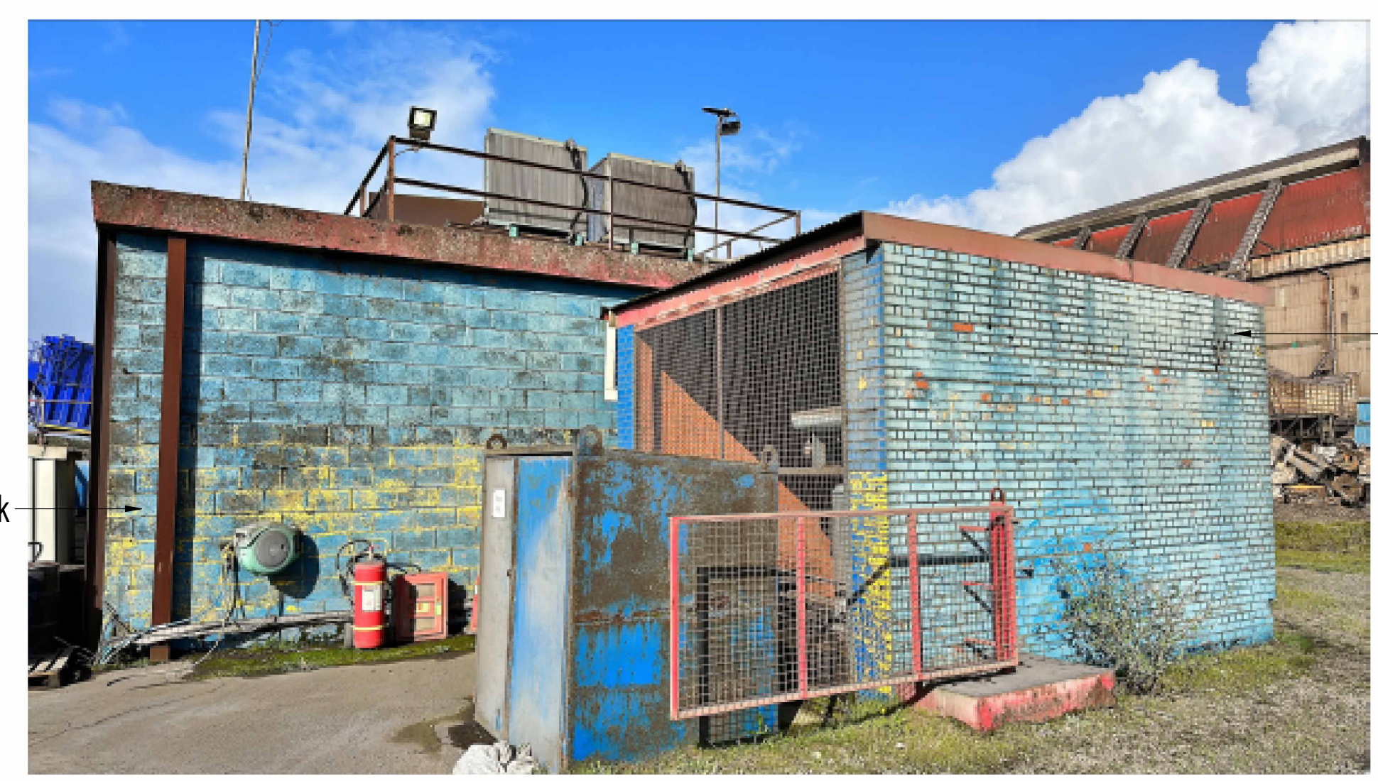
Photo 3 - Harsco Baler Plant
