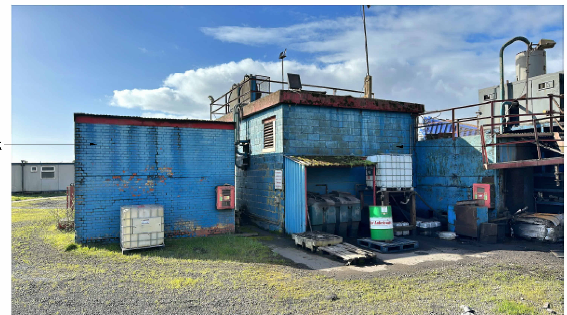
Photo 4 - Harsco Baler Plant
