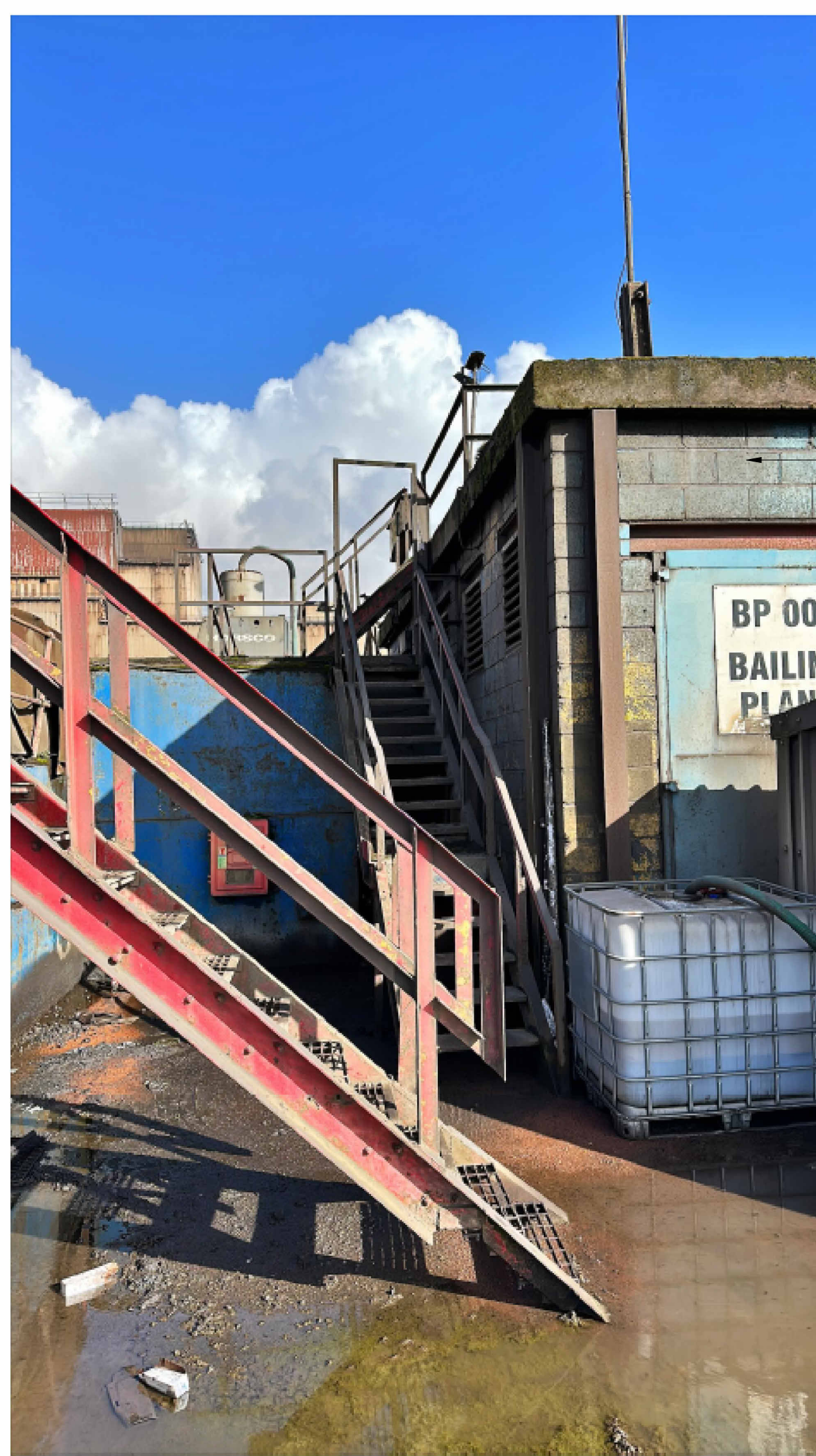
Photo 2 - Harsco Baler Plant
