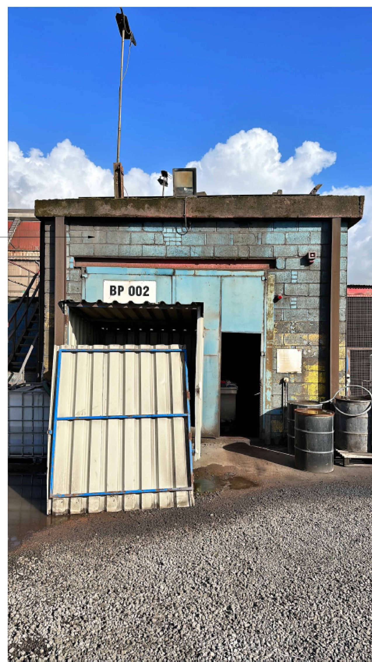
Photo 1 - Harsco Baler Plant
