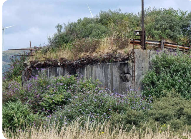
1Q Concrete Abutments
