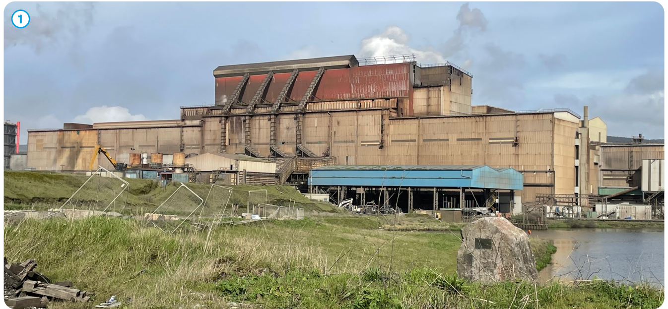
Figure 5: Distant view of the Basic Oxygen Steel (BOS) making plant
