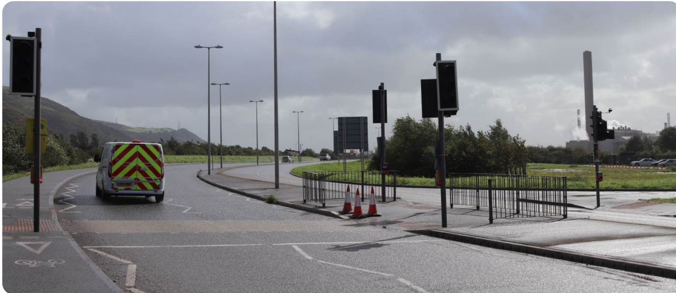
Figure 49: Pedestrian crossing on Harbour Way
