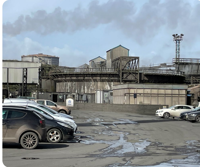
Figure 33: Parking adjacent to the BOS Plant
