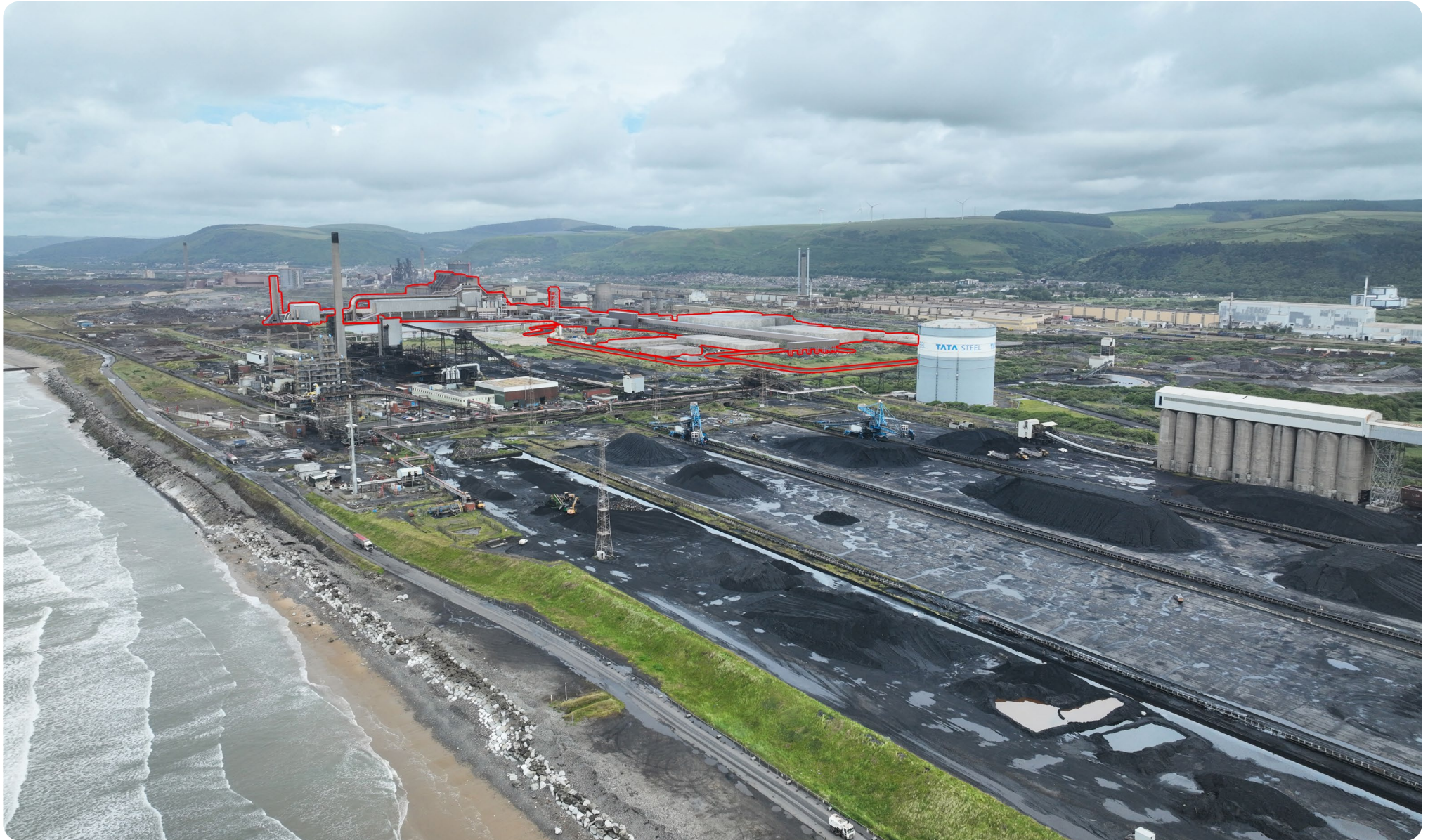
Figure 70: Indicative View of Proposals. Images are under development and will be finalised before planning application submission
