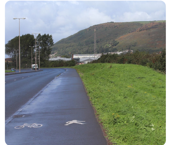
Figure 50: Shared foot/cycle way on Harbour Way
