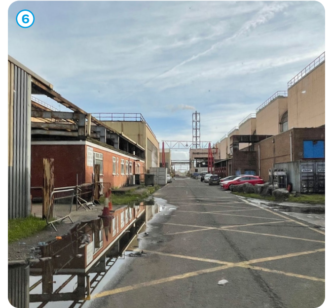
Figure 10: View between the hot and cold rolling mills
