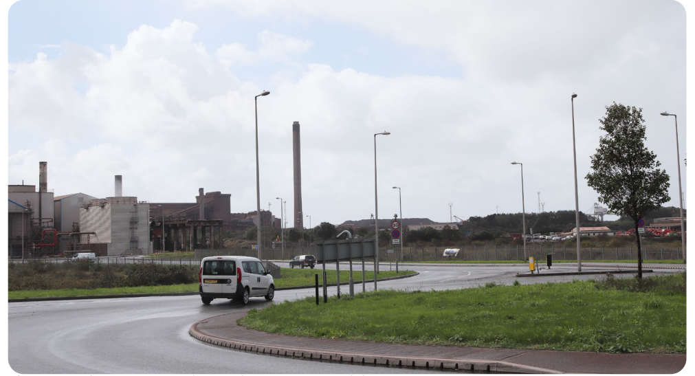
Figure 48: Site access road at Harbour Way roundabout
