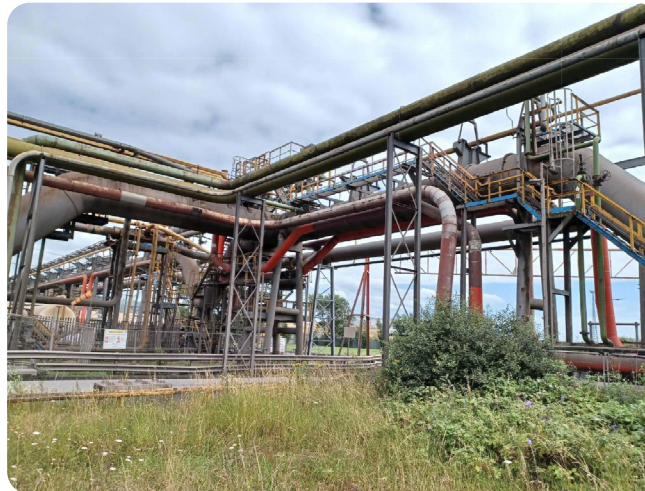
1P BF Gas Pipe Rack (Partially Removed)
