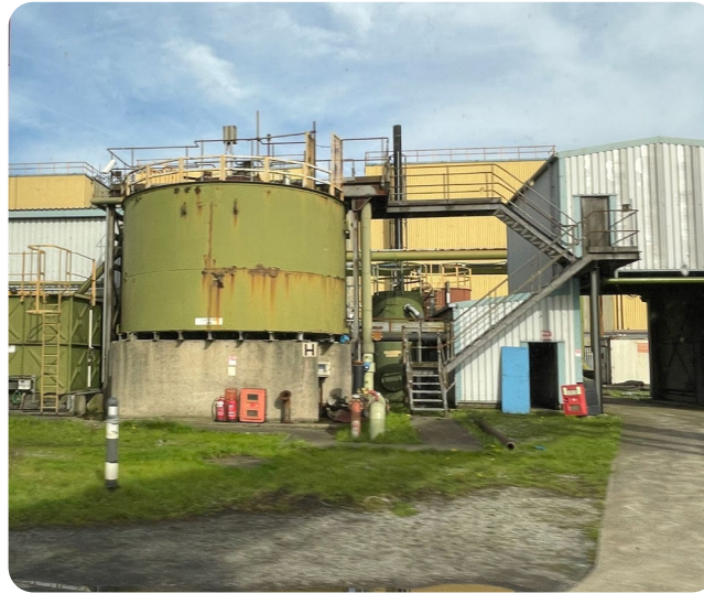
Figure 37: Rolling Mill Exterior
