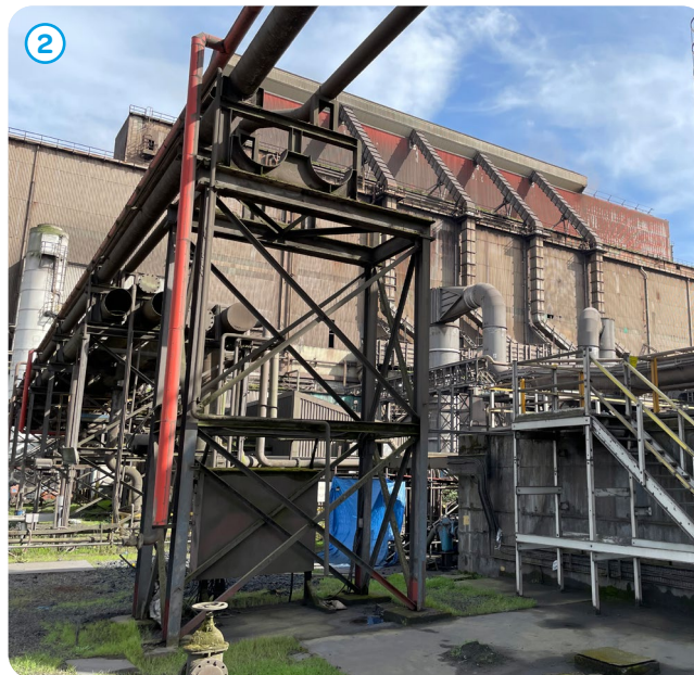
Figure 6: Close-up view of the BOS making plant
