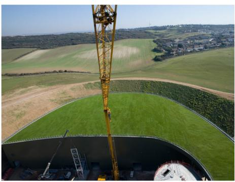
Prater Ltd has installed the UK's largest green roof of its kind at a new wastewater treatment works in Peacehaven.
