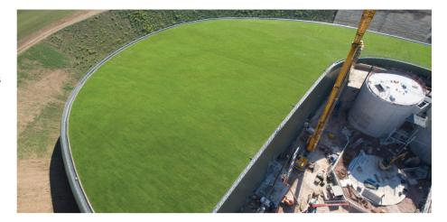
The green roof has been installed over 18,000m<sup>2</sup> of Tata Steel RoofDek D100 in Olive Green double-sided 0.9mm Colorcoat HPS200 Ultra®.
