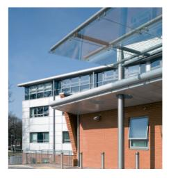
The installations are controlled and monitored by an intelligent Building Management System. A major contributor to the sustainability of the building was the specification of a TrimoRaster composite cladding system for the prominent façade areas.
