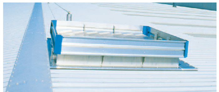
A penetration in roof cladding.
